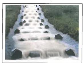
A dissipation "chute" will allow varied flows to be received and higher energy volumes dissipated as well as constrained to prevent erosion.
